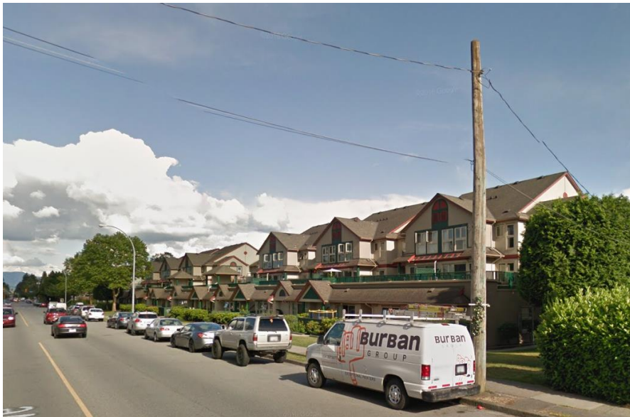
Figure 2: A large apartment development on the south side of Prairie Avenue. This example illustrates an onsite underground services connecting via a feeder line to a power pole near the property boundary.
